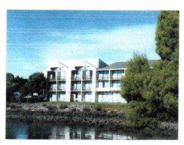
Built over a former landfill, the hotel was as close as 20 feet from the bay. Over the years differential settlement had caused cracking of floor tiles, racking of doors and window frames, separation between cabinets and walls, and roof runoff to enter the building.
